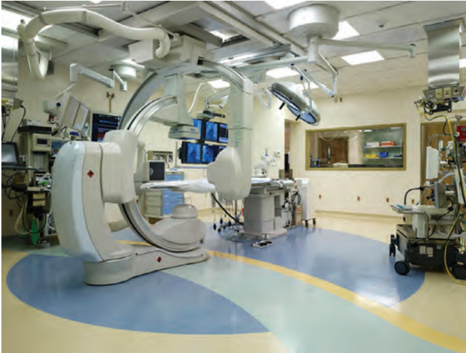
Fig. 27.1 View of a hybrid cardiovascular operating room. The cardiopulmonary bypass circuit is on the far right with its own boom. The operating table is in the middle of the picture, with a floor mounted, fixed biplanar C-arm to the left. (Courtesy of Alfred I. Dupont Hospital for Children.)
