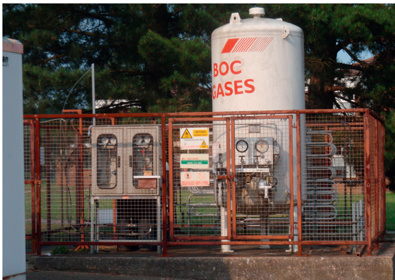
Fig. 1.20 A vacuum-insulated evaporator (VIE).
