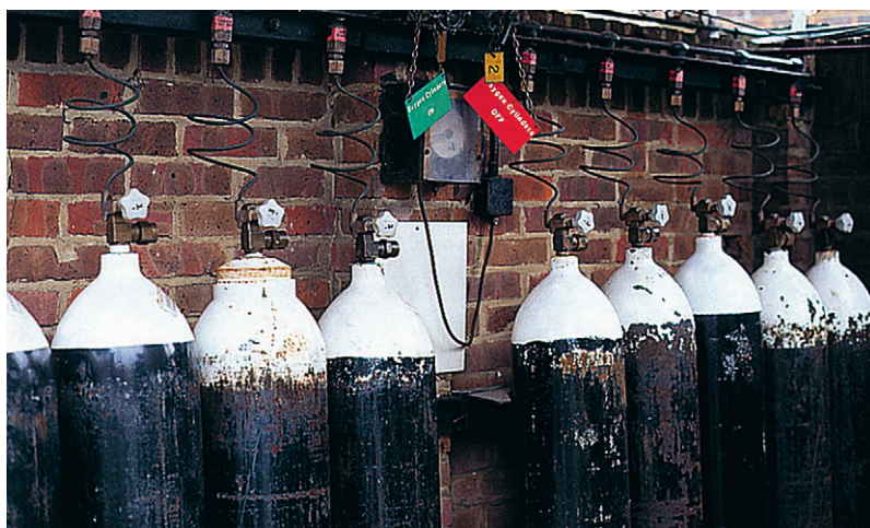
Fig. 1.19 An oxygen cylinder manifold.
