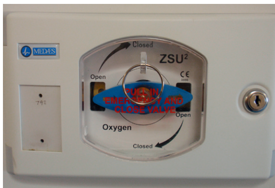
Fig. 1.16 An area valve service unit (AVSU).
